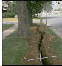
Trenching can cause significant root damage and tree death
